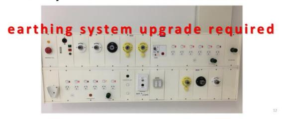
If the EP junction cannot be located or identified, the earthing system shall be upgraded to the current standard.
