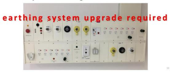
If the EP junction is being relocated, the earthing system shall be upgraded to the current standard.
