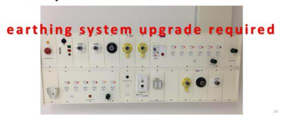
If the EP junction is inaccessible for new connections, the earthing system shall be upgraded to the current standard.
