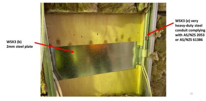
Mechanical protection at a minimum of WSX3 (refer Table H5.4 AS/NZS 3000):
