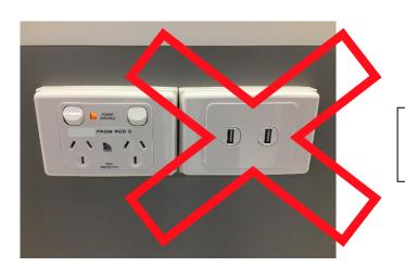
Incorrect, the USB sockets shall have a DP isolator on the 240V side of the power supplies.
