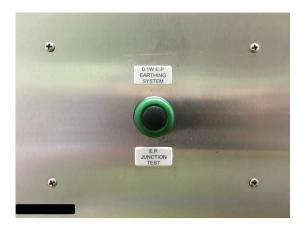
**CL.4.4.2.9** – (cardiac bonding) If the EPJ is not readily accessible, a test facility shall be provided in the cardiac-protected electrical area.
