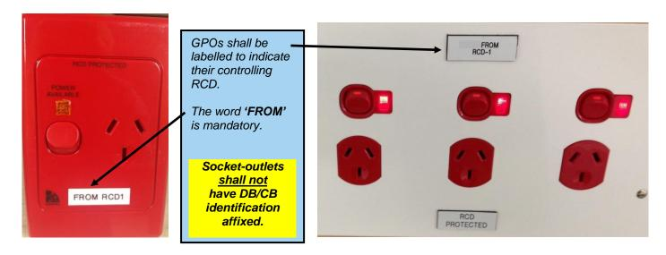
CL.2.7.4.1 – (socket-outlets) socket-outlets on RCD protected supplies (including 5m rule) shall be:
