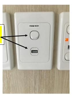
CL.2.4.3.2.2(b) – (socket-outlets) <u>2m RULE</u> – GPOs within 2m of a body protected area and are accessible without the use of a key or tool are to be RCD protected. (RCD shall be 10mA double pole).
