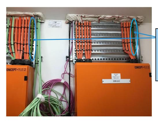
Multiple cardiac protected electrical areas and their associated EP junctions, individually connected back to their controlling switch boards via return earths.
