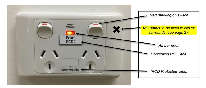
CL.2.7.4.3.1 – (socket-outlets) Colour coding of socket-outlets as follows (for 10A, 15A, 20A and ELV):
