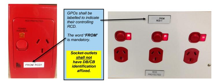
CL.2.7.4.1 – (socket-outlets) socket-outlets on RCD protected supplies (including 2m rule) shall be:
