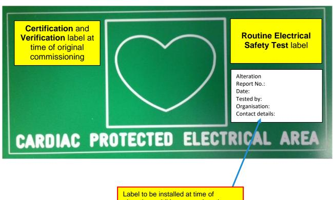
Label to be installed at time of alteration, addition or repair to the cardiac-protected electrical area.
