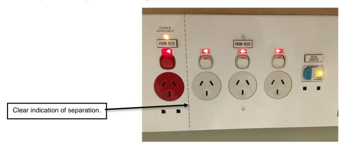
**CL.2.4.3.2.2(c)** – (socket-outlets) GPOs in ceiling spaces or imaging control rooms to be protected if supplying medical electrical equipment used within the patient area.
