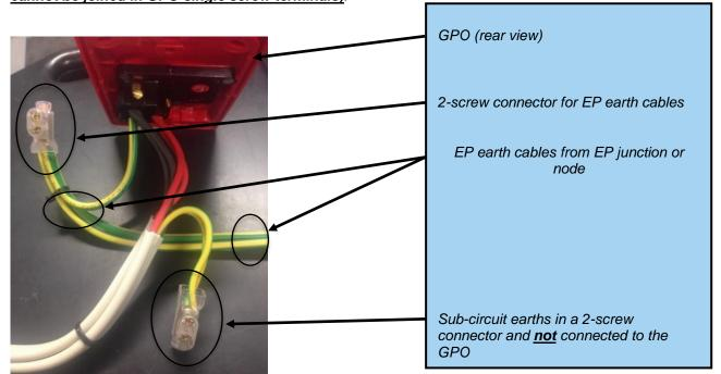
CL.4.4.2.8 - (cardiac bonding) Where the EPJ is readily accessible within the area it shall be identified -
