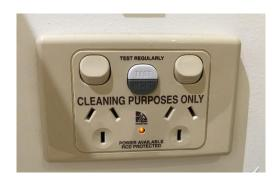
CL.2.7.3.1(a) – (cleaner GPO) Body protected electrical area – one placed within the area or within 15m of the area (see drawing page 12).
