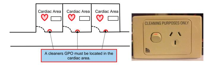
**CL.1.5.12** – (socket-outlets) Groups of socket-outlets must have clear delineation (e.g. stainless steel medical panel with a combination of different GPO supplies, an engraved line between GPO services or clear separation for easy user understanding).
