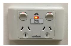
CL.2.4.3.1.2 – ELV charging socket-outlets shall be RCD protected, including USB charging socket-outlets.
