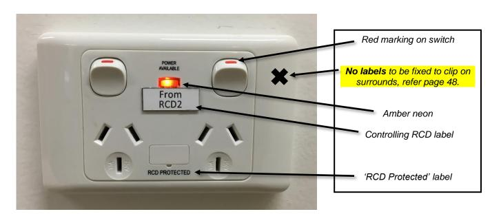
CL.2.7.4.3.1 – (socket-outlets) Colour coding of socket-outlets as follows (for 10A, 15A and 20A and ELV):
