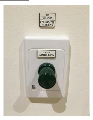
**CL.4.4.3** – (cardiac bonding) The EPJ shall be connected by return earths to each switchboard associated with the cardiac area from which the circuits originate i.e. –
