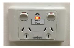
CL.2.6 (a) - (RCDs) Readily accessible and no more than 2m above the floor.
