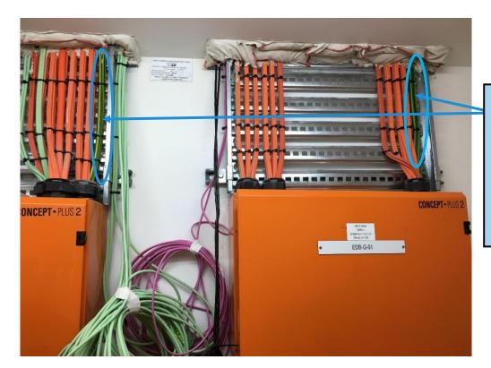
Multiple cardiac protected electrical areas and their associated EP junctions, individually connected back to their controlling switch boards via return earths.
