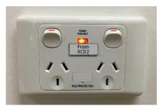
CL.2.4.3.1.2 – ELV charging socket-outlets shall be RCD protected, including USB charging socket-outlets.
