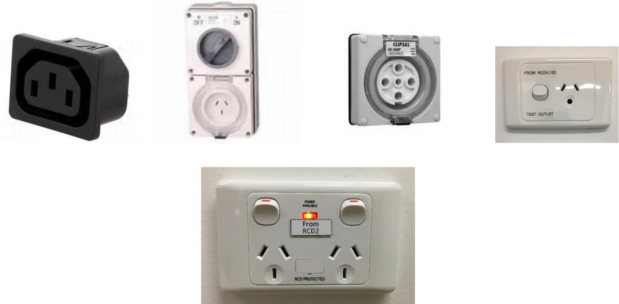
**CL.2.6 (a)** – (RCDs) Readily accessible and no more than 2m above the floor.
