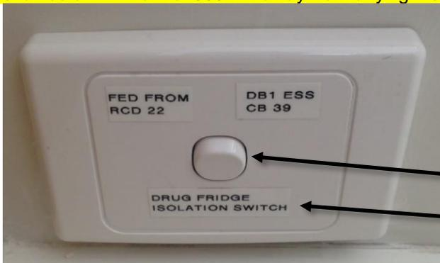
**CL. 2.10** – where permanently wired electrical equipment is supplied from an RCD that also supplies socket-outlets or other equipment, the electrical equipment shall be provided with a separate, individual, readily accessible double pole isolation switch. Not readily accessible GPOs shall be treated in the same manner.
