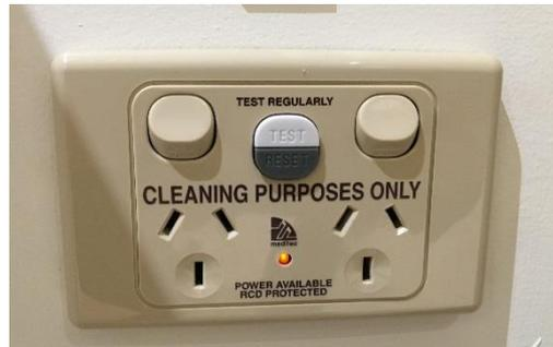
**CL.2.7.3.1(a)** – (cleaner GPO) Body protected electrical area – one placed within the area or within 15m of the area (see drawing page 8).
