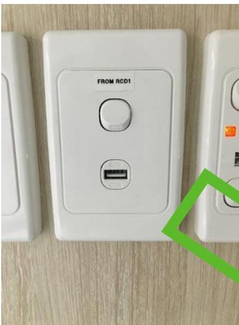
Correct, a DP isolator is incorporated into the plate to enable isolation of the USB power supply.
