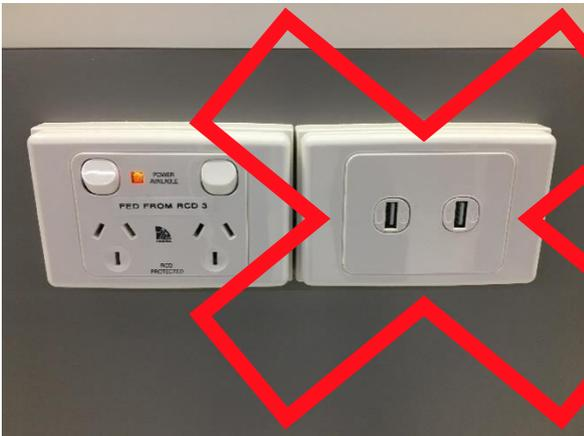
Incorrect, the USB sockets shall have a DP isolator on the 240V side of the power supplies.
