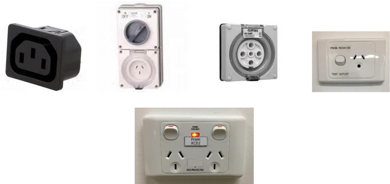
**CL.2.6 (a)** – (RCDs) Readily accessible and no more than 2m above the floor.
